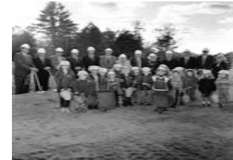
Big and Small Dignitaries on Groundbreaking Day
